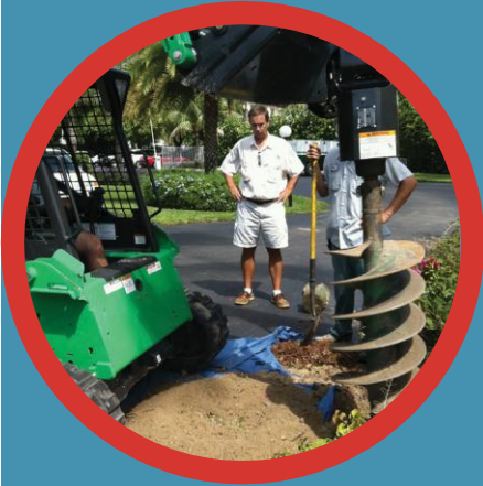
Holes are dug for new lighting.
