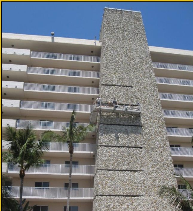
Repairs to the stone facade are complete.
