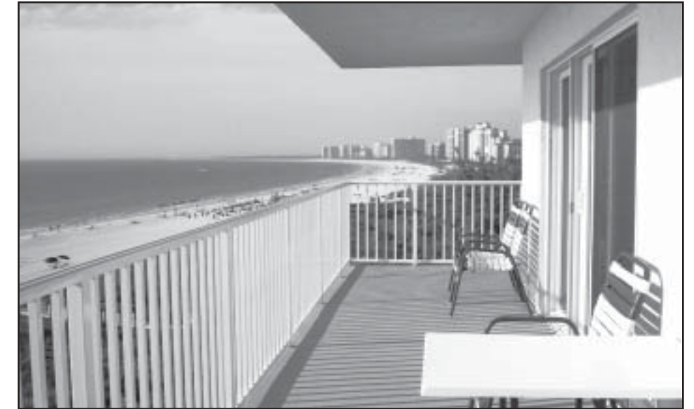
The new balconies and railing look beautiful. The balconies were taken down to bare concrete. New railing was installed on all unit balconies.
