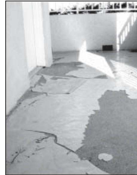
Resurfacing of The Hurricane Wilma-ravaged walkways begins in May.
